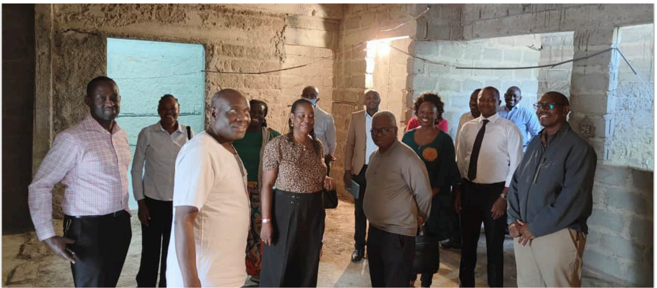
Kisumu building and renovation project site visit
